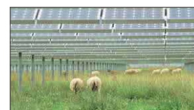
Farm solar generation system
