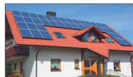
Off-grid home solar system
