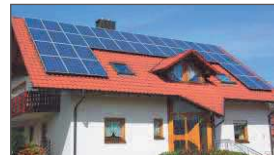
Off-grid home solar system
